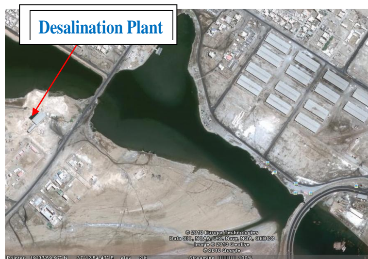
Figure (1) : Desalination Plant – Sea Land lagoon
